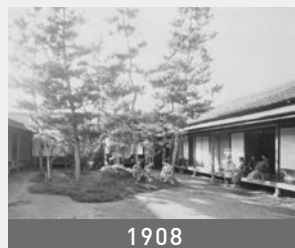
Detached family housing units
